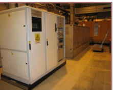
100kV solid state modulator for LINAC 4 at SM18 hall at CERN. Design, developed and Commissioned by RRCAAT.
